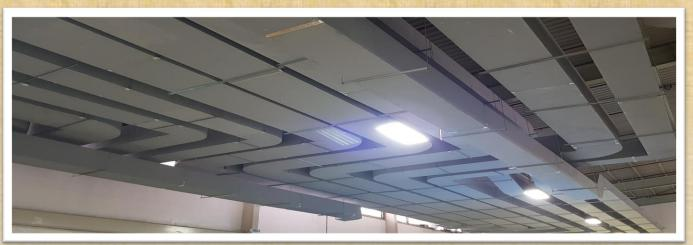
Thermal conductivity is 0.022 W/m°C with no mechanical joins on the longitudinal duct section. Therefore is thermally better and very minimal leakage compare to conventional duct system.
