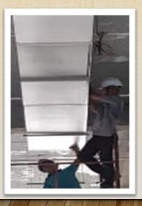
TDM duct is very light weight, 6 times lighter than G.I. duct with insulation. This significantly reduced building load, roofing load and ceiling load. Also it uses less hanger, less labour and faster installation time. Suitable for commercial office buildings, factories and malls.
