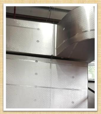
TDM Pre-insulated aluminium duct is developed as an alternative to the conventional ducting system. It is a sandwiched panel made of PIR (POLYISOCYANURATE) foam covered in smooth or embossed 80 micron aluminium foil (anti-mould & anti bacterial coated).
